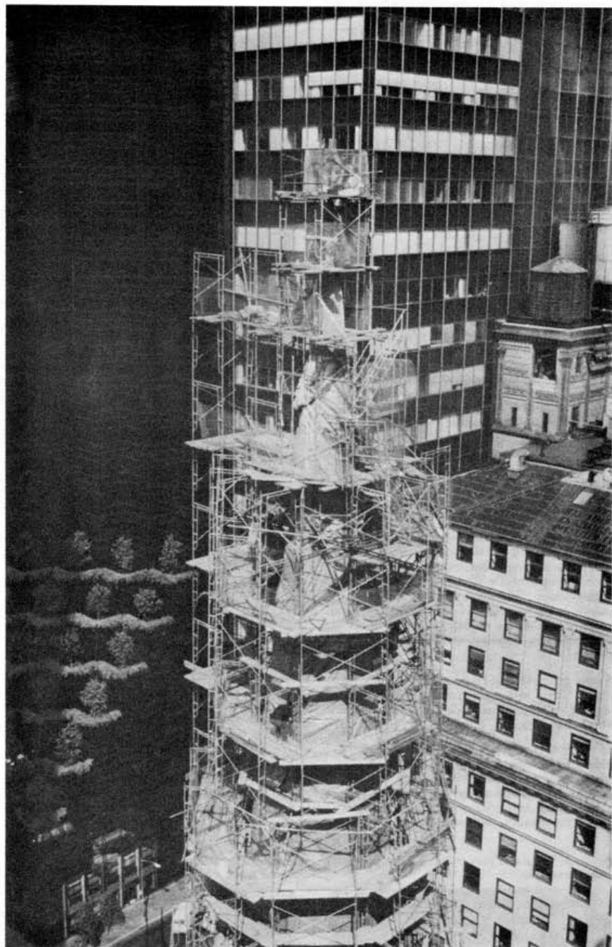
Gilding the cross atop Fifth Avenue Presbyterian Church. Cathedral Stoneworks is the principal contractor for the $3.5 million "stone-by-stone" restoration.
