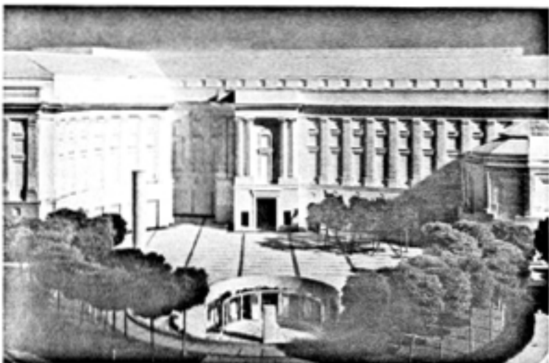
The primary cladding for the Federal Triangle Building will be Indiana limestone, while Deer Isle granite is being used for the water table.
