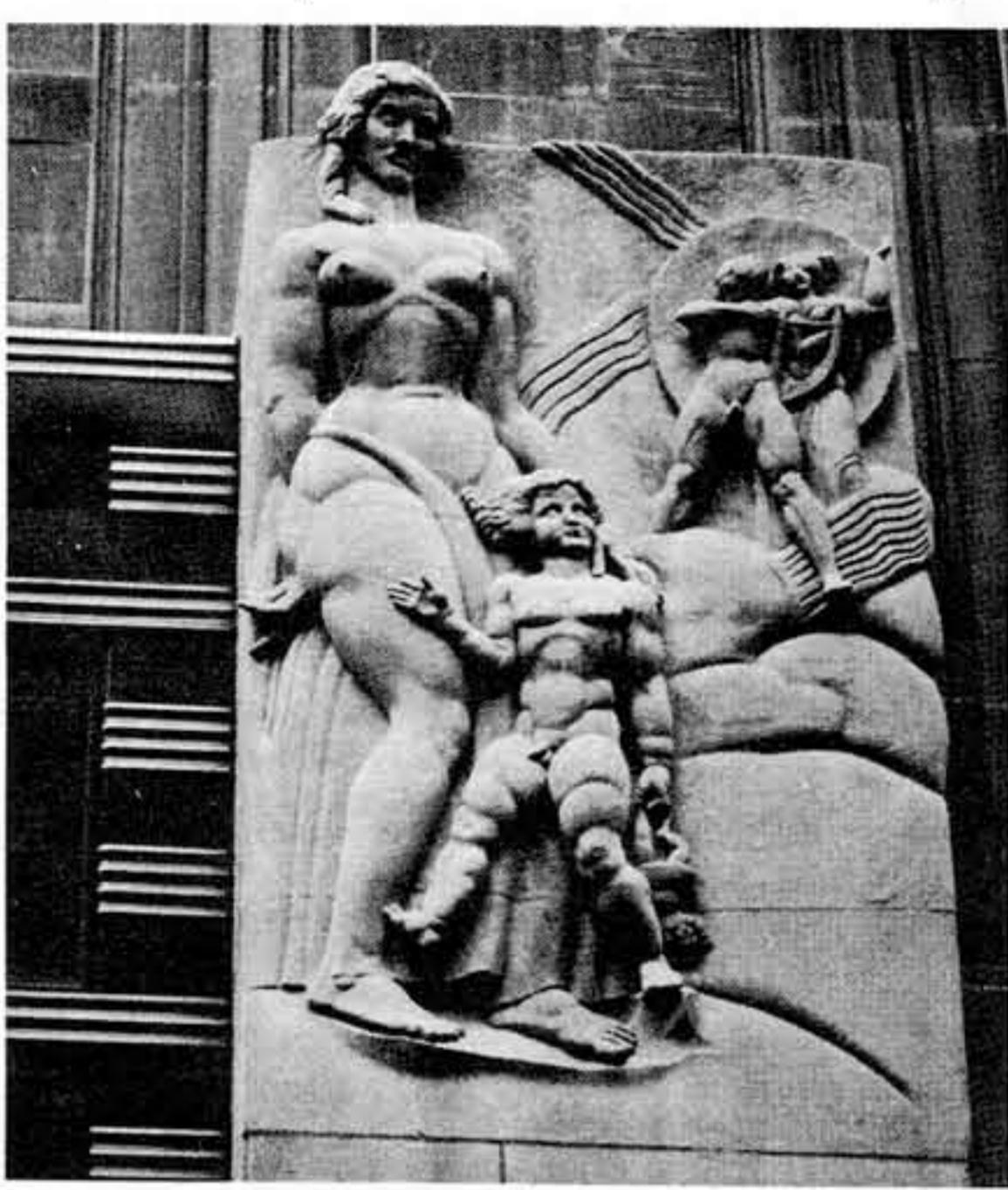
The maintenance and restoration of limestone facades on the 60-year-old Rockefeller Center include the repair of both sculptures (foreground) and thick ashlar panels (background). Photo: Cathedral Stoneworks
