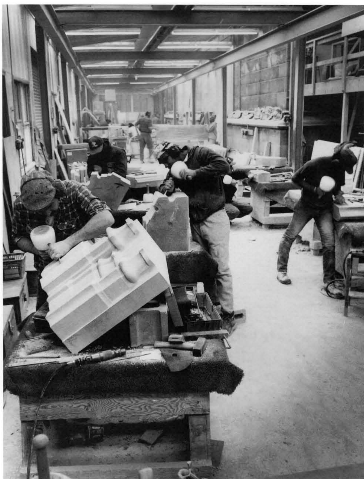
The new banker mason shed.
